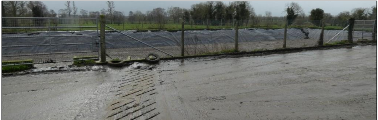
Photo 9: View looking south towards the Slurry Lagoon with intercepting slatted slurry channel taking any soiled yard drainage from the open yard and diverting this to the slurry lagoon. This is one of at least 3 of such channels
